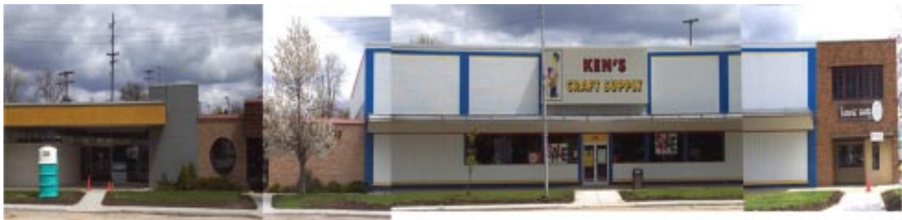
Existing conditions at east quadrant.
