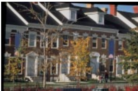
Maisonettes look very much like townhomes with entrances at street level, but have higher density because the units are stacked.
