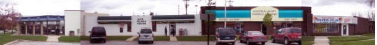
Existing conditions in northeast quadrant.
